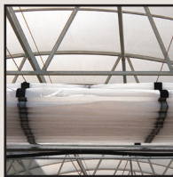
Sub Roof Fabric
